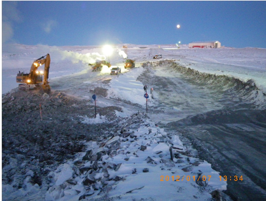
Photo 1: Snow has been removed from the keytrench. At the right of the picture, some of the 5/8" clear material has been pushed into a wind-row which will be mixed with the ROQ that will be removed from the upstream side of the keytrench and placed within the downstream footprint of the dam. Snow removal continues along the top of the ROQ surface along the downstream side of the dam, as shown at the left of the picture. Photo looking east from the west side of the keytrench.
